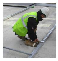
Intermediate profile beams are then laid out parallel to the eave of the structure. These create the support rails of which the floorboards are laid on. These are then adjusted to the correct width so that the runners sit up in the correct position for the board to slot into.
