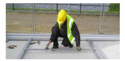
The ground surface will have imperfections and this can affect the level of the floor system. In the case of this happening the use of a laser level will detect any rise or falls in the ground. The use of metal shims brings the floor to the exact level needed to ensure the structure is of a safe standard. These are placed at the joins of the bars and at two other points along the beam to reduce flex in the intermediate profile.
